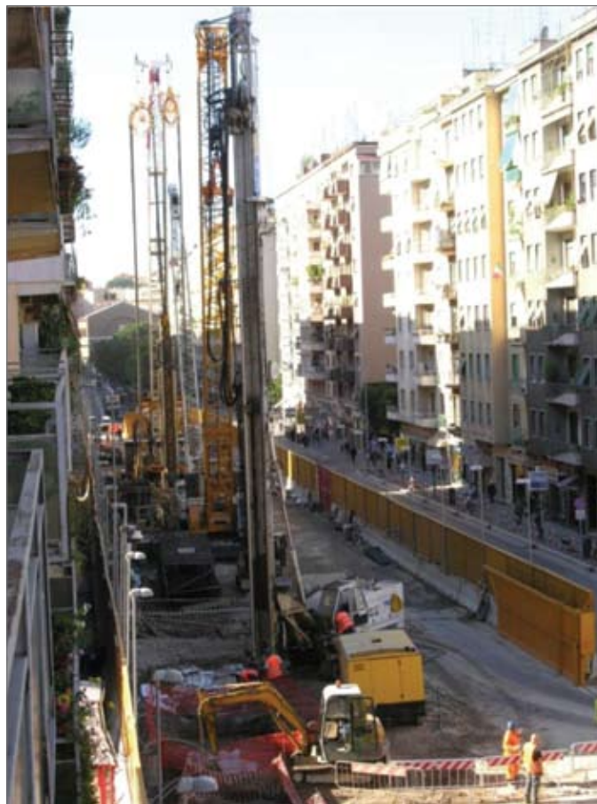
Fig. 6. City of Rome — Impact of the works
