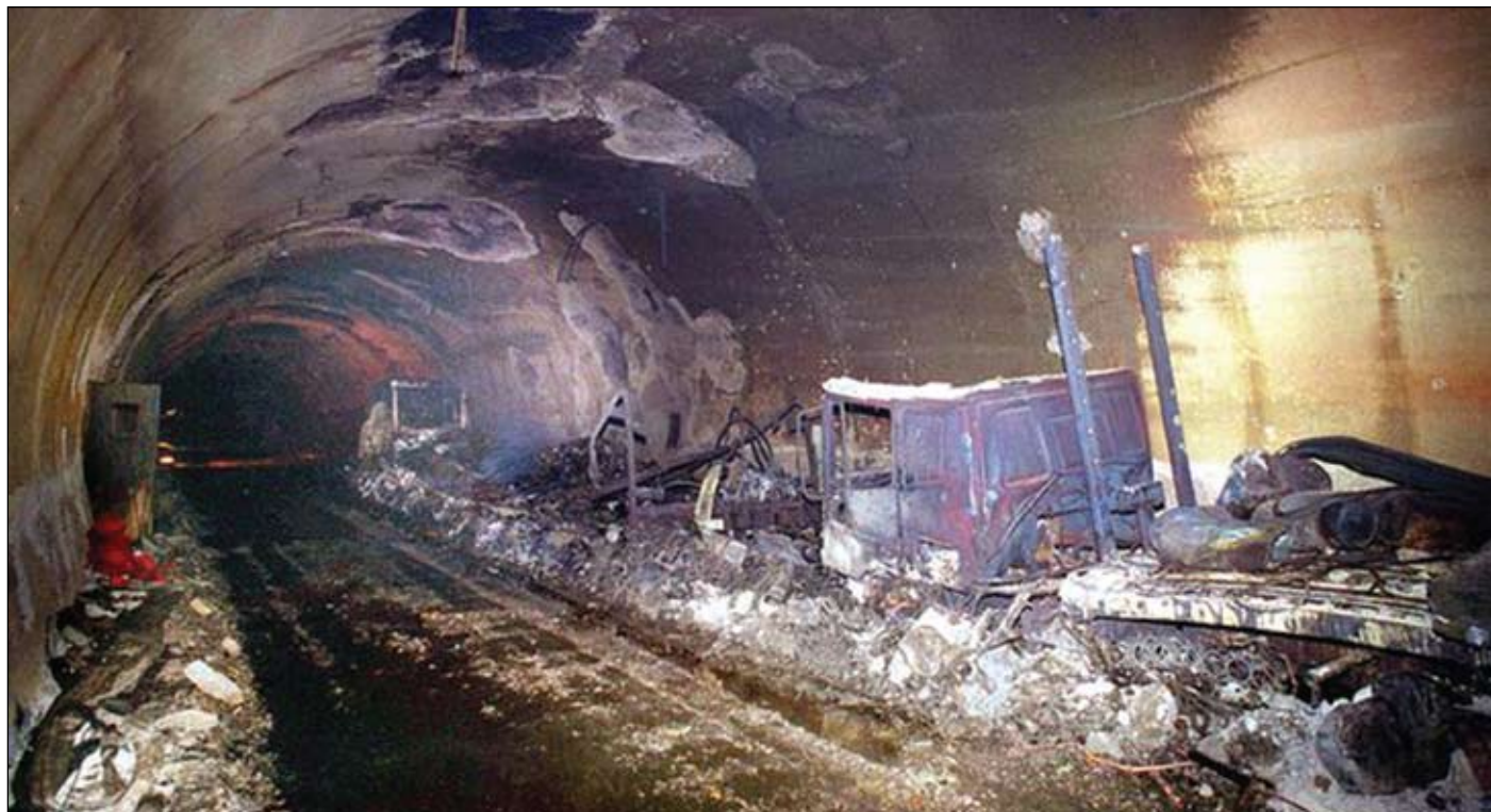
Mont Blanc tunnel, France-Italy 1999
