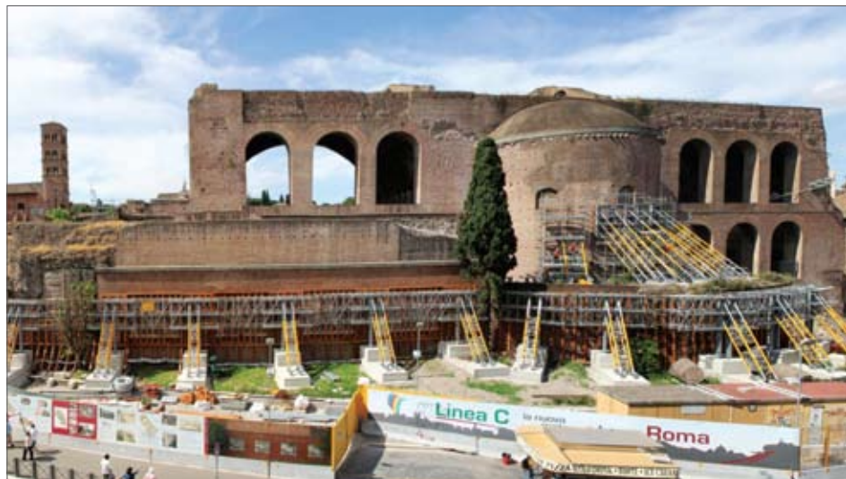
Fig. 5. The reinforcement of Basilica of Maxentius
