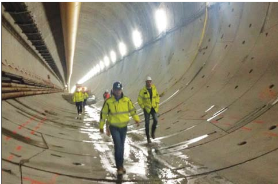
SS 640 Porto Empedocle – Galleria Caltanissetta- Italia
