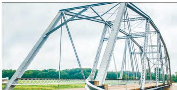
Chicago Ave Bridge
