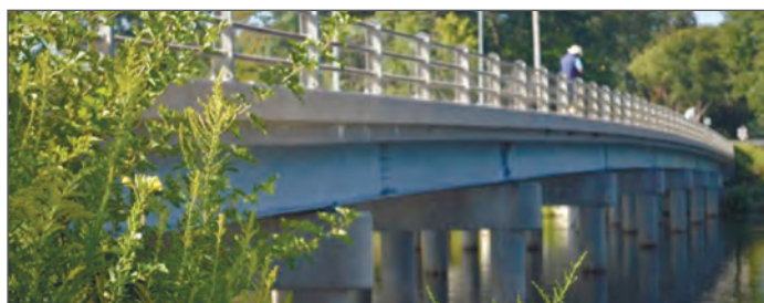
Stearns Bayou Bridge
