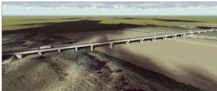
Pioneer River Bridge (AECOM Australia)
