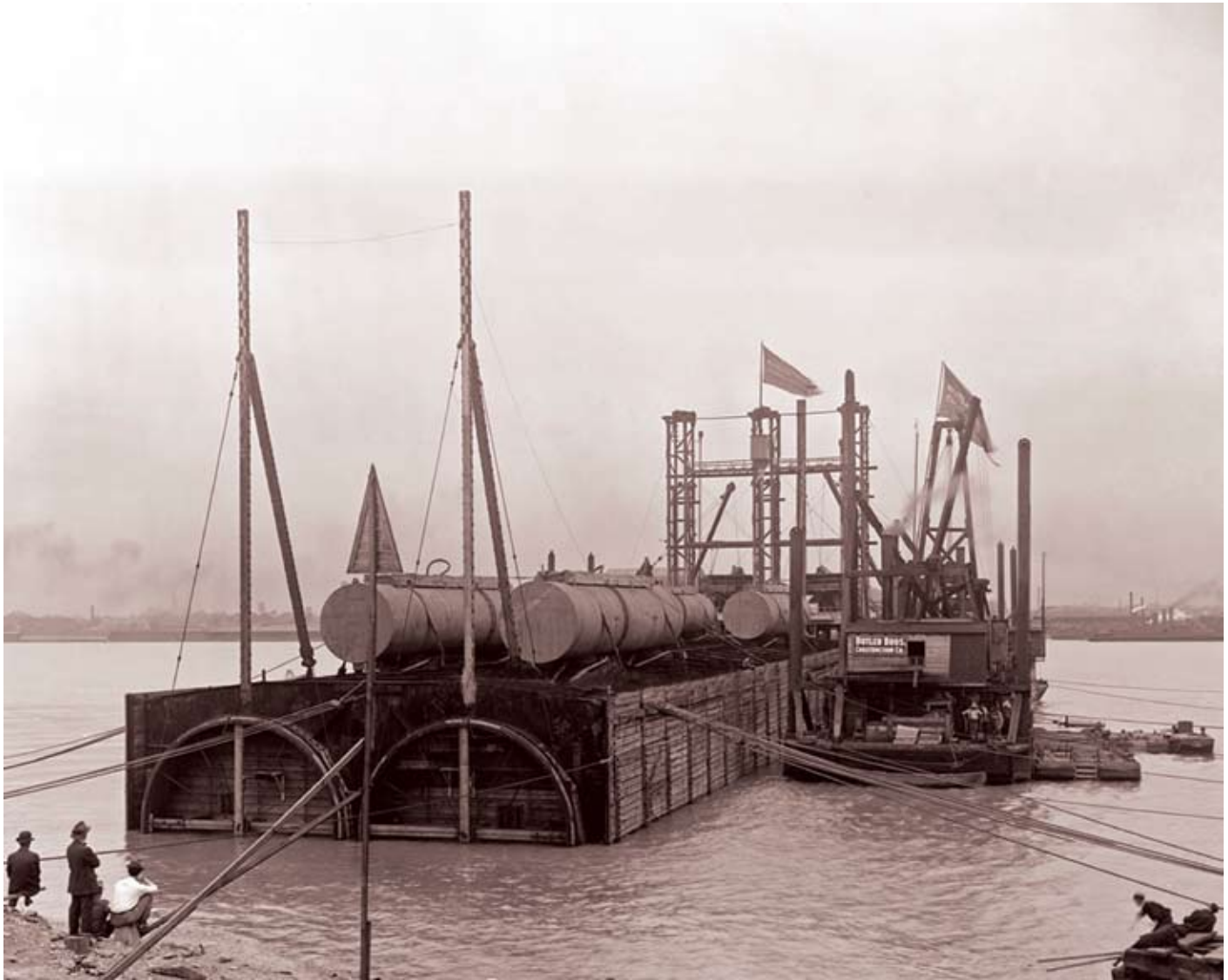
Sinking Tubular Sections, Detroit River Tunnel
